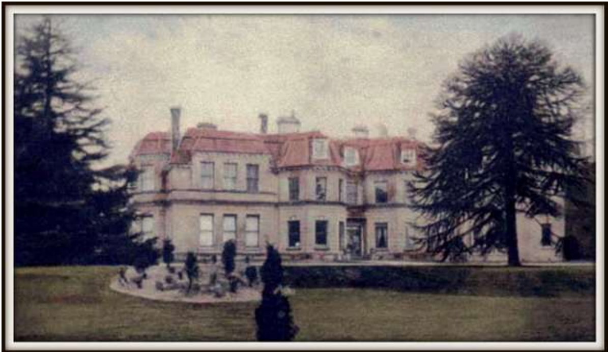
Ladham House, Kent
